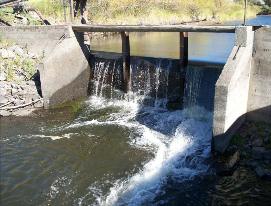
Figure 7. Photo of Diversion Structure located at station 67045 on Catherine Creek, illustrating the use of boards to increase backwater. Photo from Anderson Perry Surveys, September 28th 2010.
